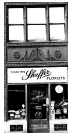
This finely detailed bronze storefront is typical of many constructed during the 1920s. The original grilles, spandrel panel and windows are all intact. Photo: NPS files.
