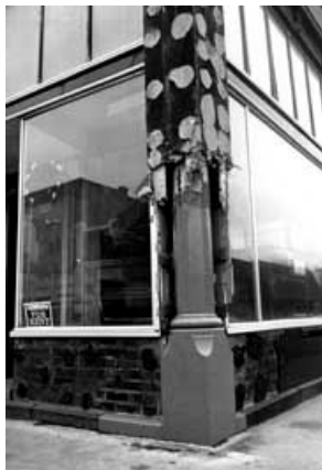
Storefronts of the 1940s, 50s, and 60s were frequently installed by attaching studs or a metal grid over an early front and applying new covering materials. Photo:
