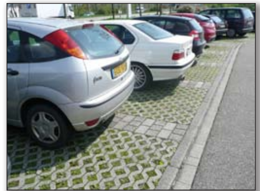
Permeable paving of parking swales.
