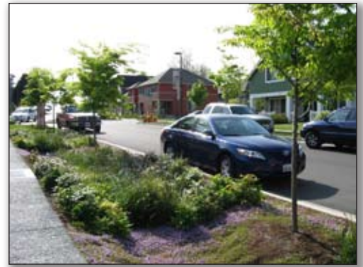
A vegetated buffer strip along a street allows infiltration of stormwater.
