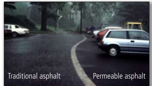
Permeable asphalt treatment of parking stalls.
