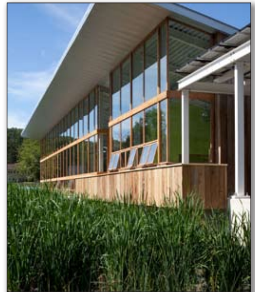
Constructed wetland wastewater treatment facility at Omega Institute in Rhinebeck.
