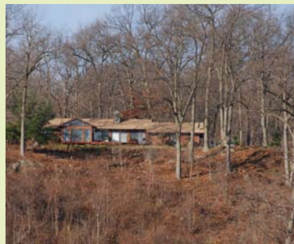
Natural building materials, dark color, and selective trimming of vegetation provides river views without creating adverse visual impact.
