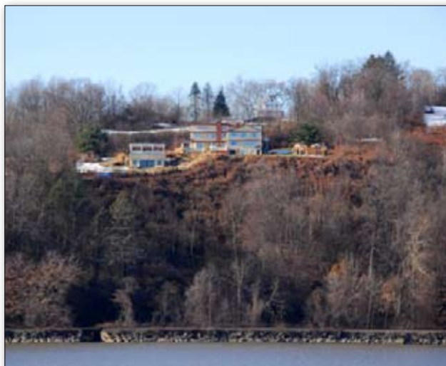
This large home, built close to the bluff line, is unscreened by vegetation and highly visible.
