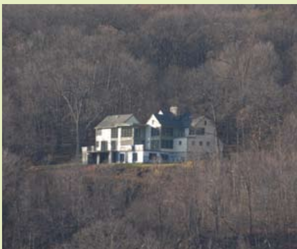
Even with provisions of Waterfront Bluffs Overlay District, this home still lies unshielded from river.
