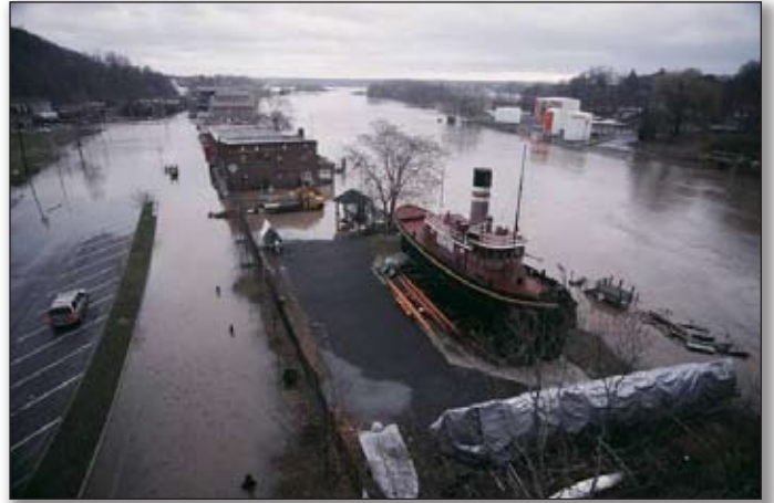
April 2005 flooding in the City of Kingston.
