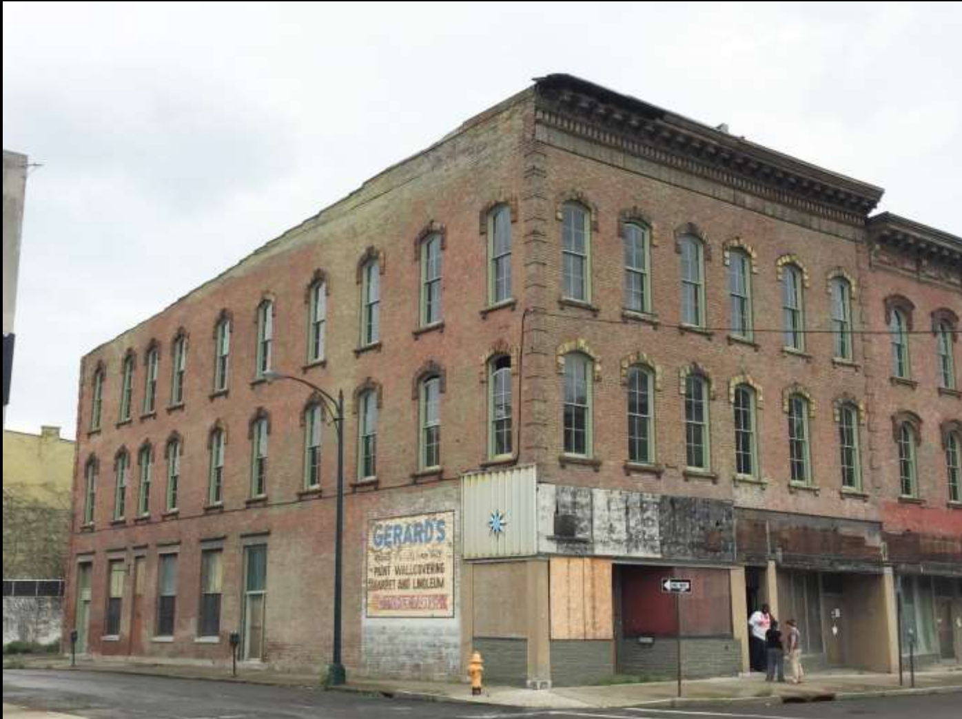
Elmira, NY Artist Housing in Construction
