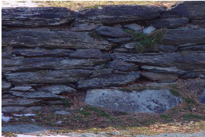
Figure 5: Close up view of Stone Wall
