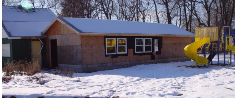
Figure 1: Community Center (under construction)
