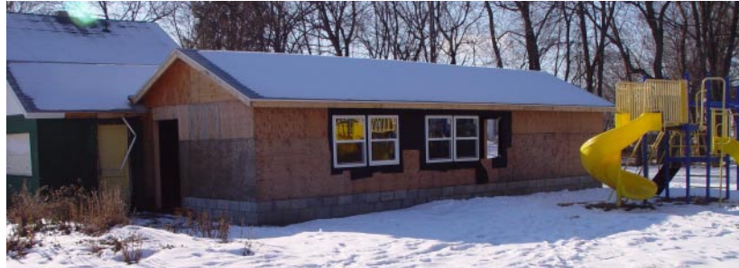
Figure 16: Summit Lake Community Center (under construction)
