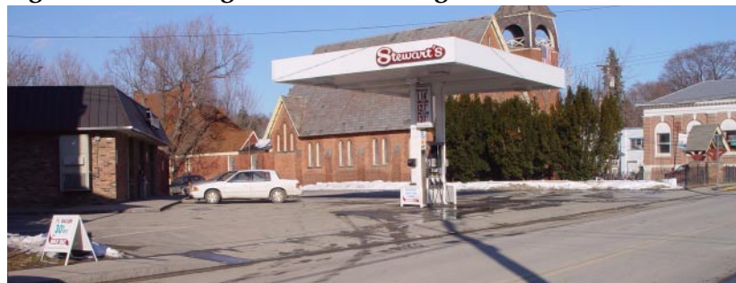
Figure 13: Parking Lot and Building Askew
