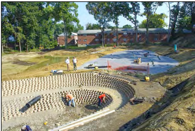
Construction of Forebay
