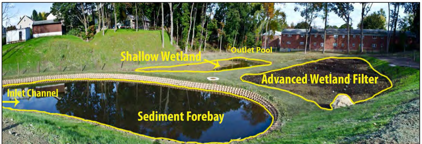
Sedimentary forebay (retention pond) in foreground, with gravel wetland filter above and outlet pool on right
