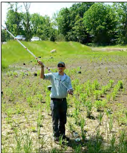
Lead Engineer David Whitney uses "sludge-judge" to demonstrate clean water coming from clean out pipes
