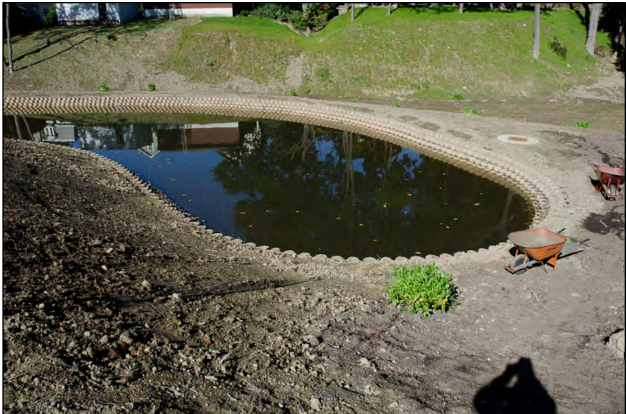
Forebay filled with stormwater
