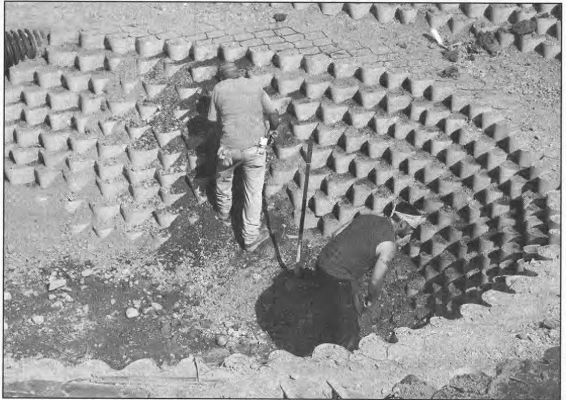
Workers put the finishing touches on the drainage project in Wappingers Falls.
