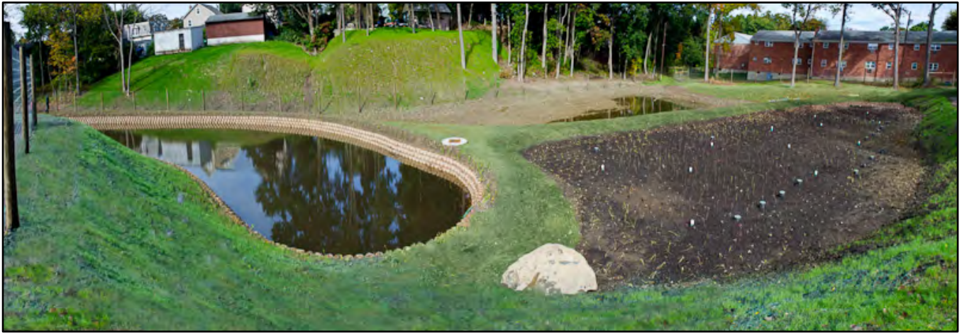
Construction Complete, site planted and landscaped – Oct. 2013
