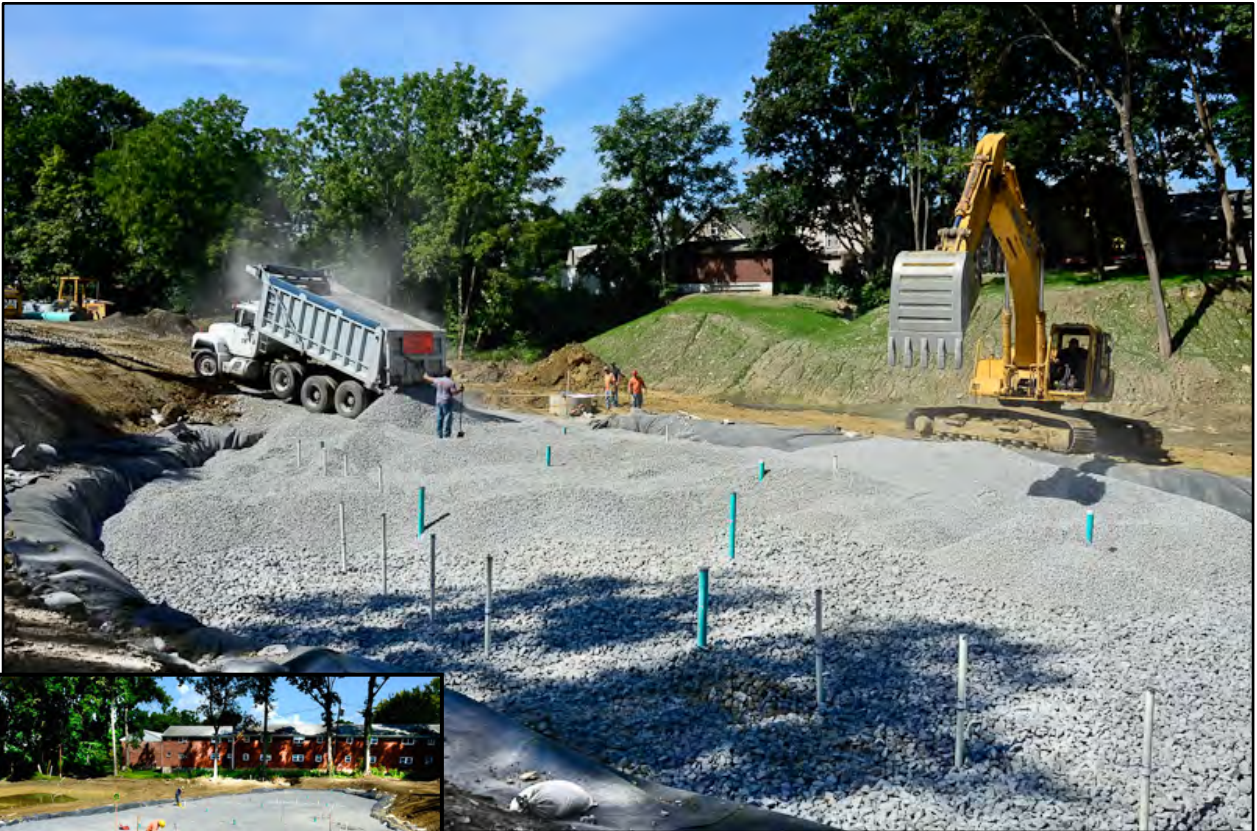
3 different size layers of gravel backfilled onto wetland August 2013
