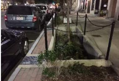
Planter boxes are urban rain gardens with vertical walls and either open or closed bottoms. They collect and absorb runoff from sidewalks, parking lots, and streets and are an ideal streetscaping element.
