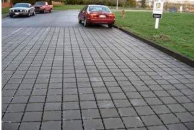
Permeable pavements infiltrate, treat, and/or store rainwater where it falls.
