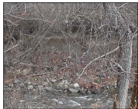
Failing Stream Bank
