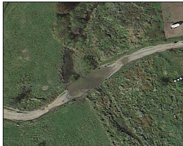
Unstabilized Stream Crossing
