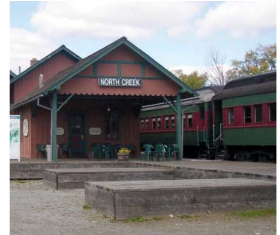
North Creek rail stop, North Creek
