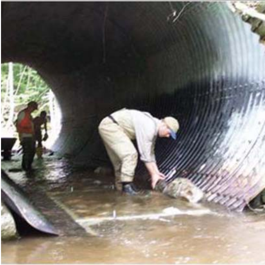
Stream barrier inspection
