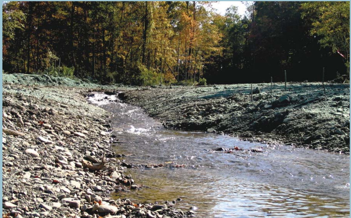
Six Mile Creek, streambank stabilization
