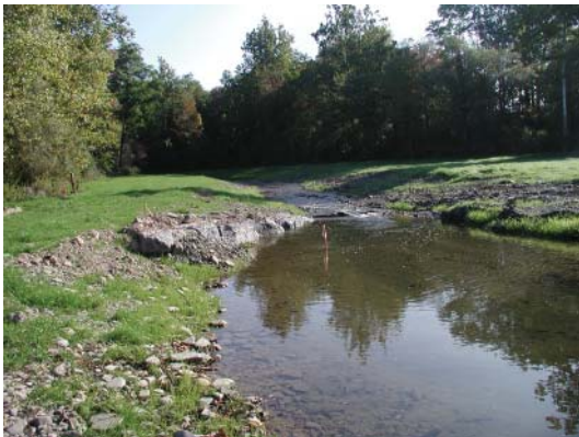
Six Mile Creek restoration, Caroline
